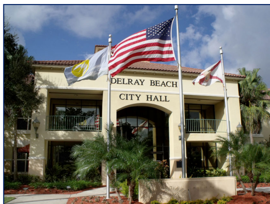
Delray Beach City Hall, 100 NW 1 st Avenue
