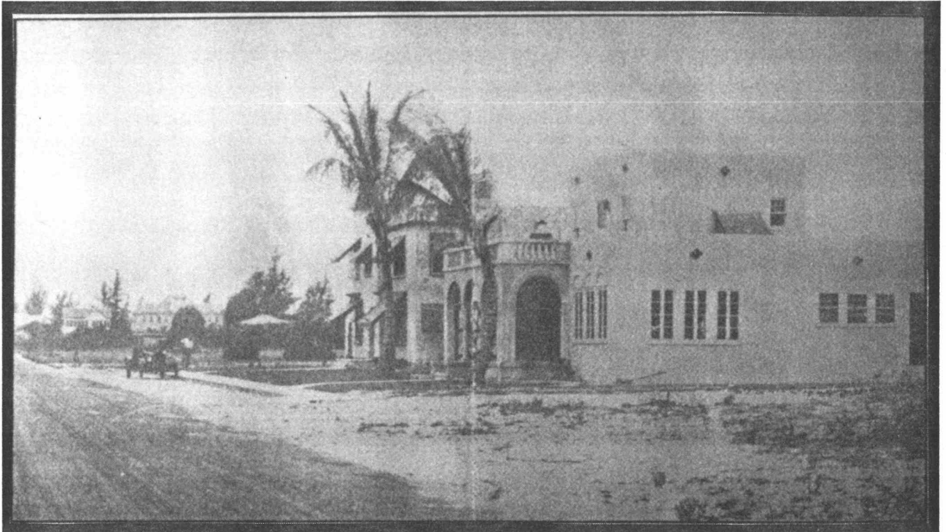
Fig. 12 Looking South L.H. Walker House Foreground (#234) J.C. Keen House (#226) 1926 Chamber of Commerce Promotional Brochure
