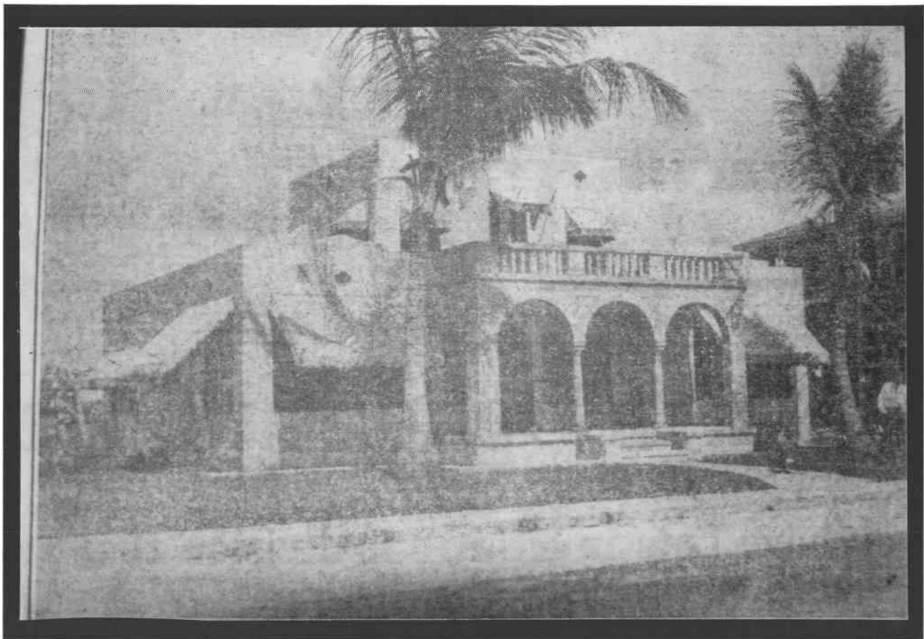
Fig. 8 L.H. Walker House (#234) Front (East) Facade The Delray News, 8/14/1925
