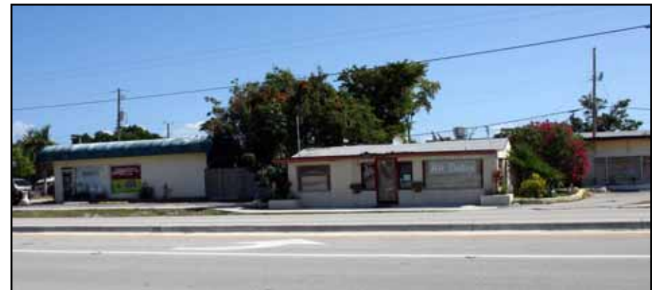
Figure 2.12 – These Dilapidated Buildings in the 2700 Block Should Be Redeveloped.
