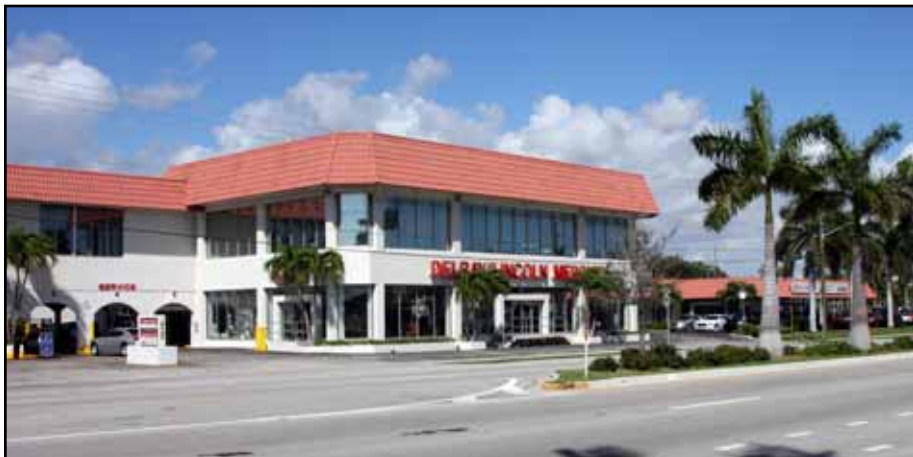
Figure 2.2 – Delray Motors - 2102 South Federal Highway
