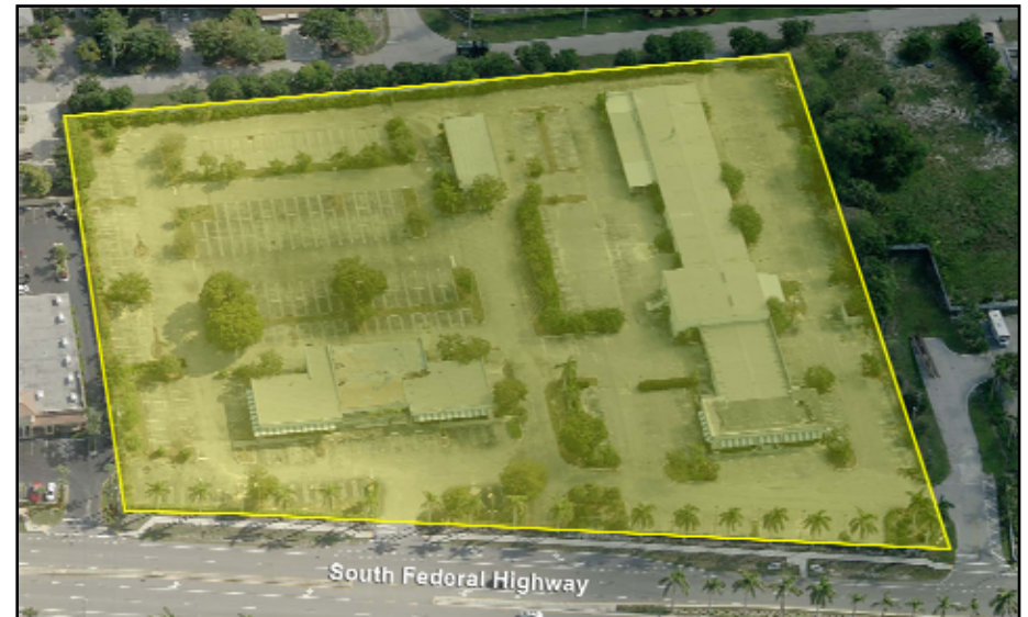
Figure 3-2 – Ralph Buick Property at 2501 South Federal Highway
