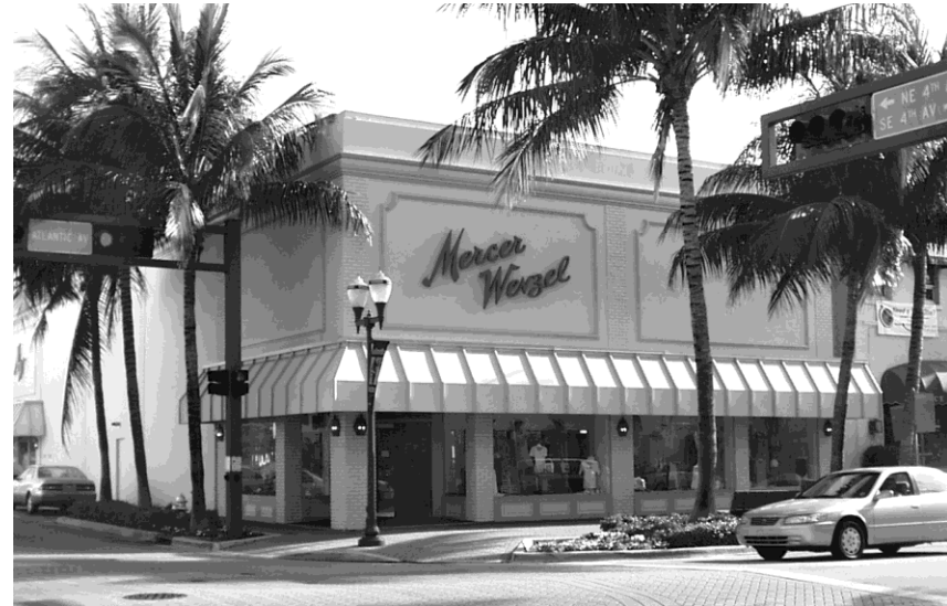
Masonry Vernacular commercial building
