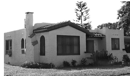
This Mission style house combines a gable roof of barrel tiles and flat roof. (Note that the chimney has elements of both the exterior surface and the roof.)
