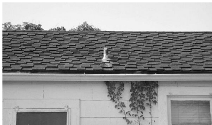
Example of irregular style roof shingles
