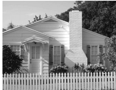
The brick chimney on this residence is
