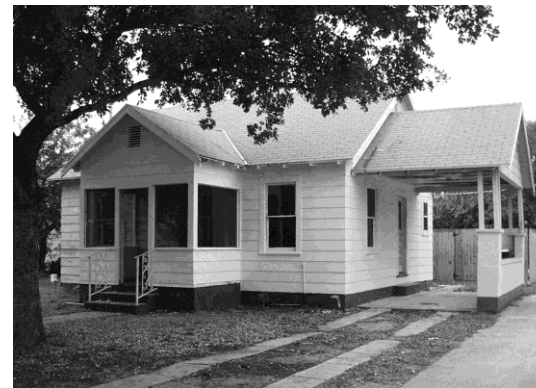
An example of weatherboard siding
