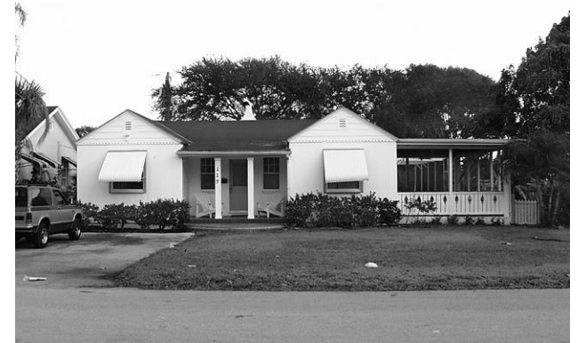
Minimal Traditional residence
