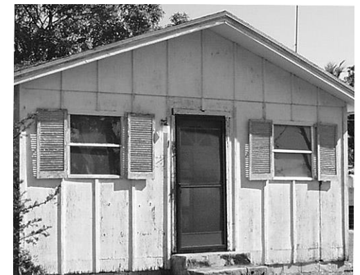
Board and batten siding
