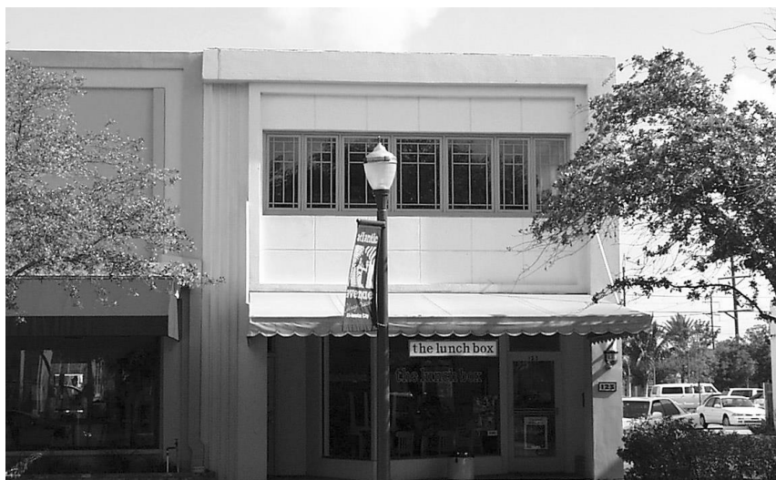
Masonry Vernacular commercial building
