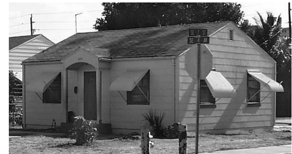
WWI-era Frame Vernacular residence
