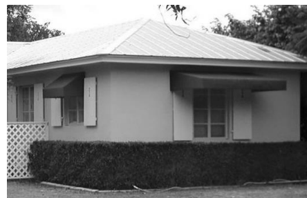
A standing seam metal, cross-hip roof
