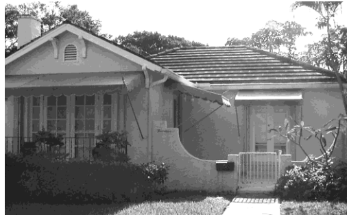
Textured stucco on masonry walls should match the textured stucco on the main building.
