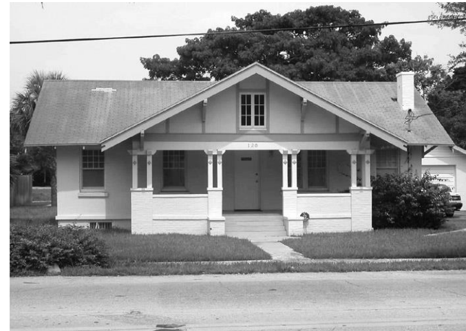
The exterior of this residence is a combination of stucco and painted brick.
