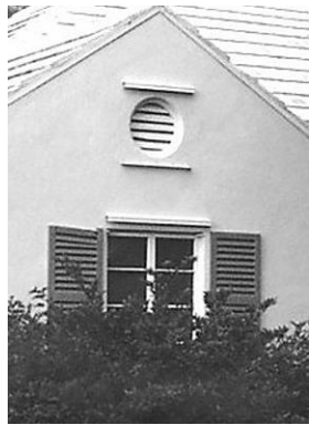
Track installed year-round should be painted to match the building.
