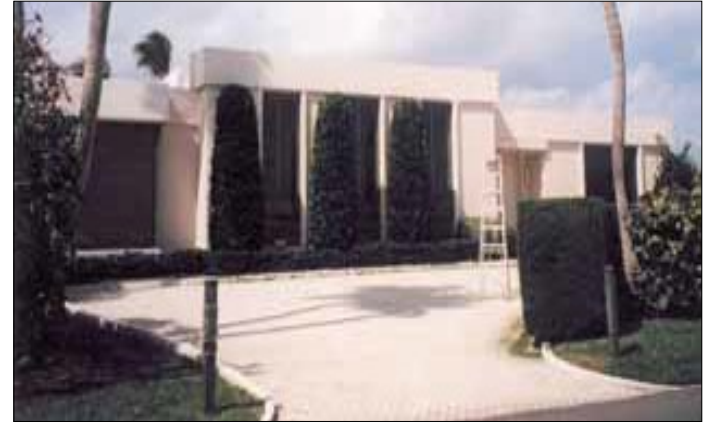
Regency can take on a commercial office or even a governmental appearance. (Additional Review Required)
