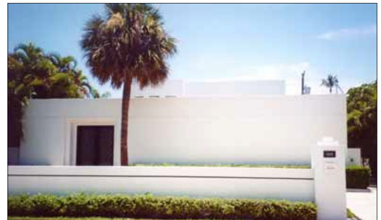
Prohibited: Unarticulated blank/flat wall over 16' long on front facade
