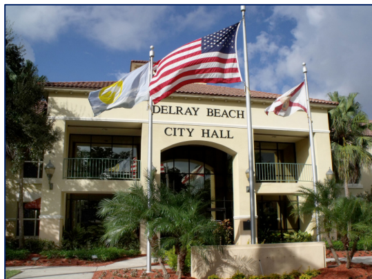
Delray Beach City Hall, 100 NW 1 st Avenue
