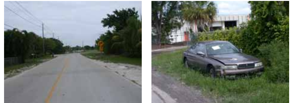
Figure 14 – Existing Right-of ways within the Redevelopment Area
