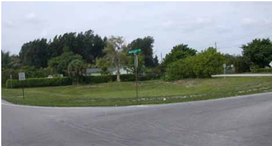
Figure 15 – Existing Storm Water Detention Area
