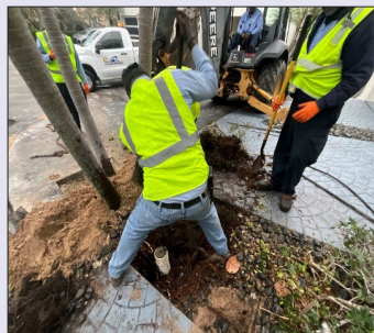
2115 S Ocean Blvd Leak Repair
