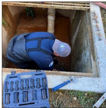
Clearing drain lines
