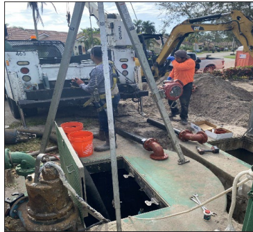
Lift Station 93A rehab
