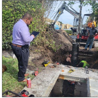
Monitoring contractor installation of 8" backflow prevention device assembly
