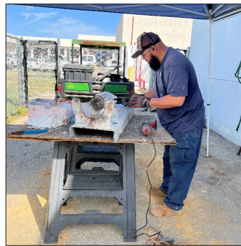
Rehabbing the lime slurry pumps
