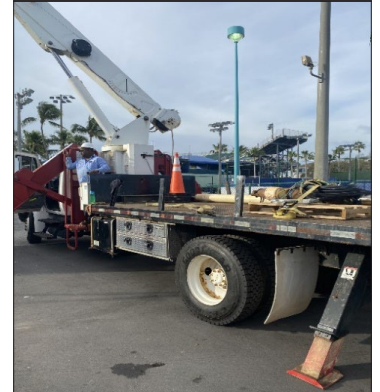
RWW 6 pump replacement
