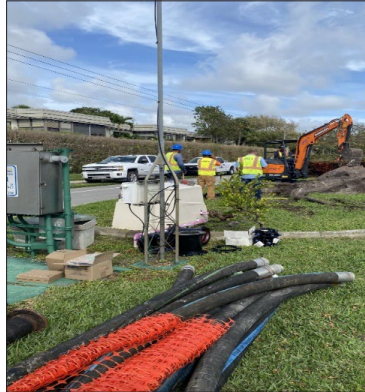
Lift Station 51 repairs
