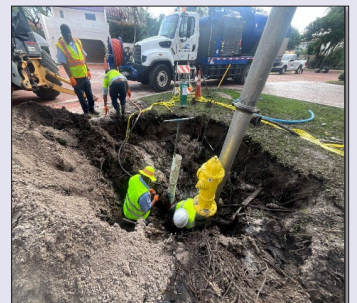
3578 Commodore Circle Hydrant Replacement
