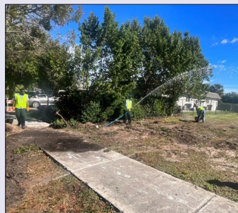
S. Swinton Ave. Service Line Replacement
