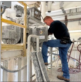
Inspecting the lime slakers
