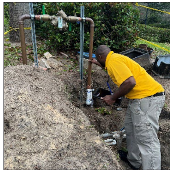
Inspecting pipe composition
