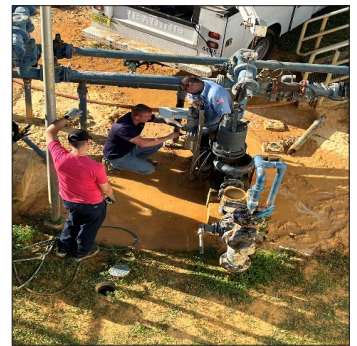
Installing and testing sludge pumps
