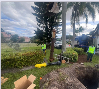
Sherwood Blvd. Hydrant Replacement
