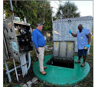
Lift Station 60 pump replacement
