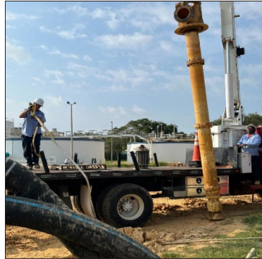
Recovery basin pump installation
