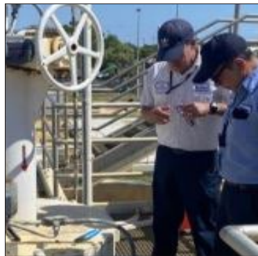
East thickeners repairs
