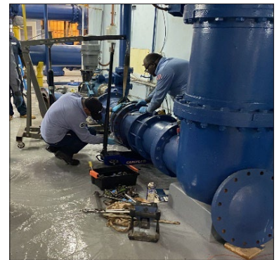
Filter 2 actuator installation
