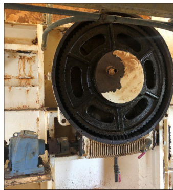
Vacuum Filters Repairs
