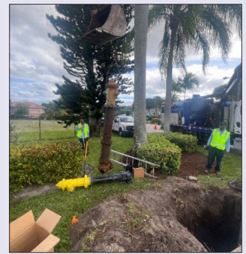
Sherwood Blvd. Hydrant Replacement
