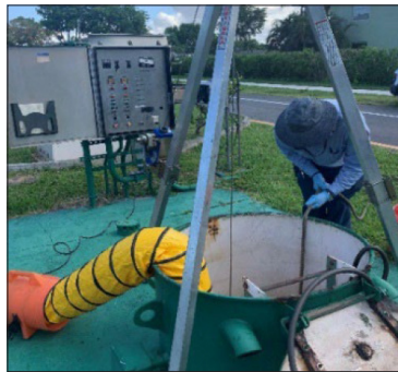
Lift Station 51 Repairs
