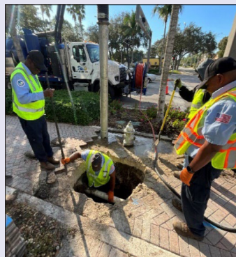
Fire Hydrant Replacement W. Atlantic Blvd.
