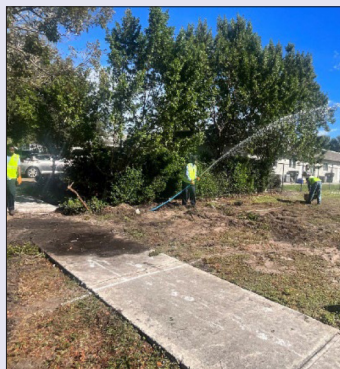
S. Swinton Ave. Service Line Replacement
