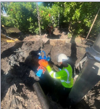
Valve Replacement N. Ocean Blvd.
