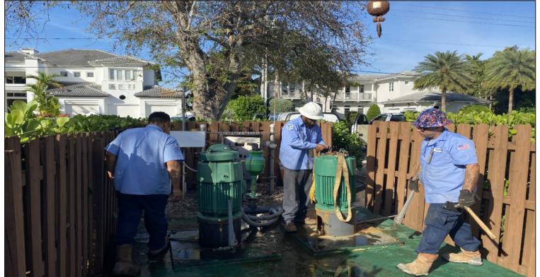
Seasage Storm Station Repair
