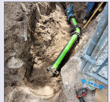
Contractor installing new forcemain at Lift Station 086
