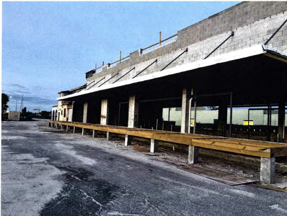
Exterior Site Photo 2
