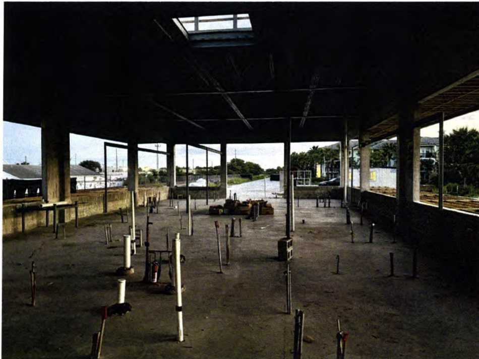
Interior Site Photo 2
