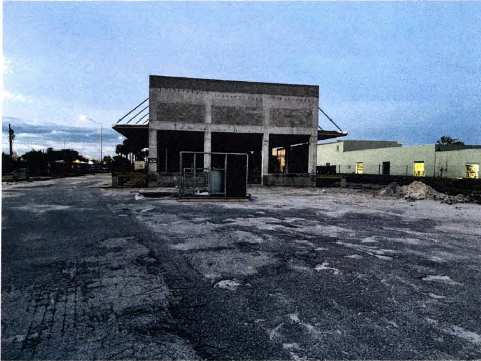
Exterior Site Photo 1
