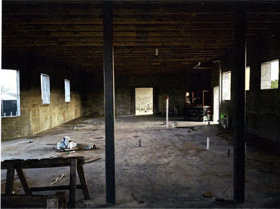
Interior Site Photo 1
