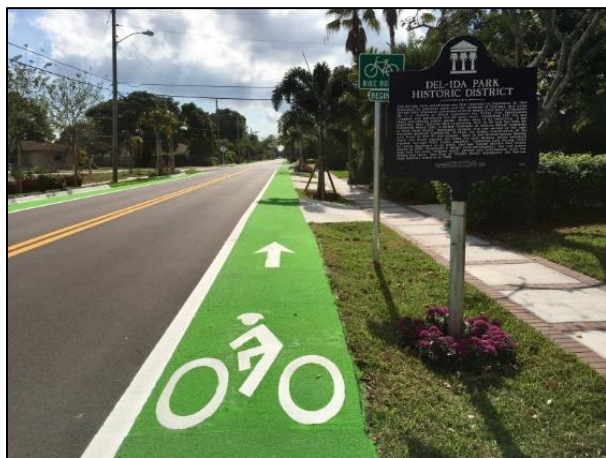
NE 2 nd Avenue Improvements Source: spbc.blog.palmbeachpost.com
