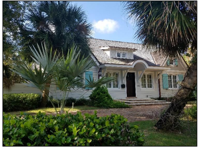
Waters-Wellenbrink Residence; 1108 Vista Del Mar Drive
