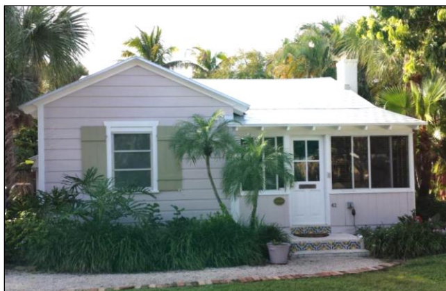
42 Palm Square; the property owner utilized the Income Tax Credit Program to assist in the improvements to this contributing structure.
