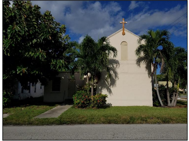
St. Matthew Episcopal Church; 404 SW 3 rd Street
