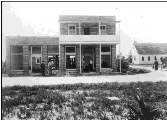
4 East Atlantic Avenue; Circa 1910 Oldest Existing Commercial Building on Atlantic Avenue
