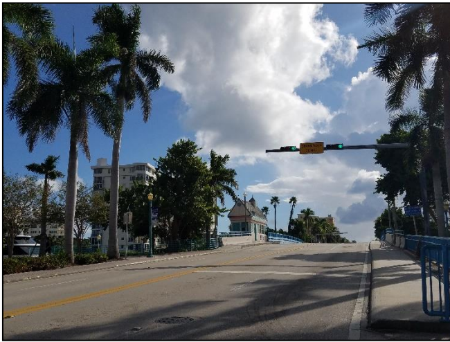
The Atlantic Avenue Bridge
