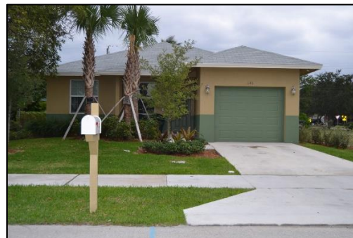
Single Family Home constructed by Habitat for Humanity of South Palm Beach
