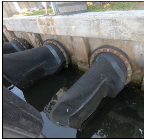
Duckbill Installed - Courtesy of APTIM 2018
