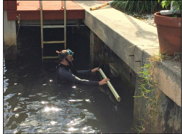
APTIM Performing Outfall Inspections - Spring 2018
